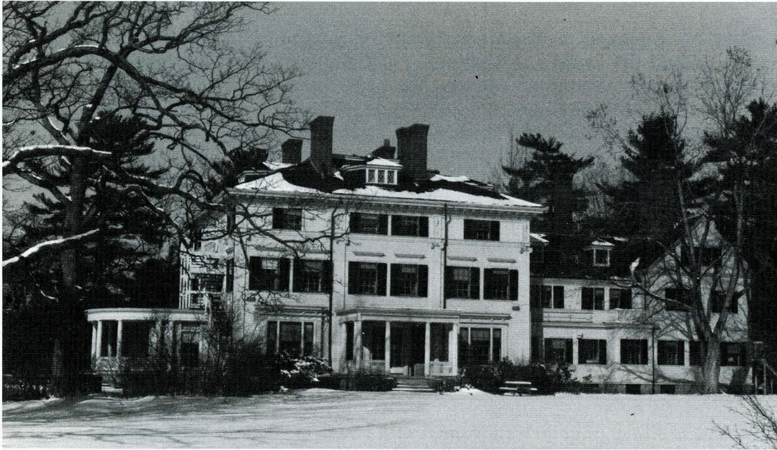
Cheever House, site of the Wellesley College Center for Research on Women
